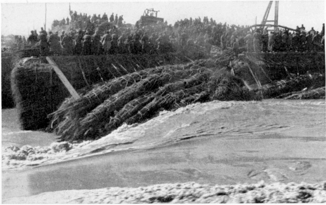
FIG. 8—Closing the final gap in the 5000-foot-wide break at Huayuankou by use of long willow-stone “sausages.”
