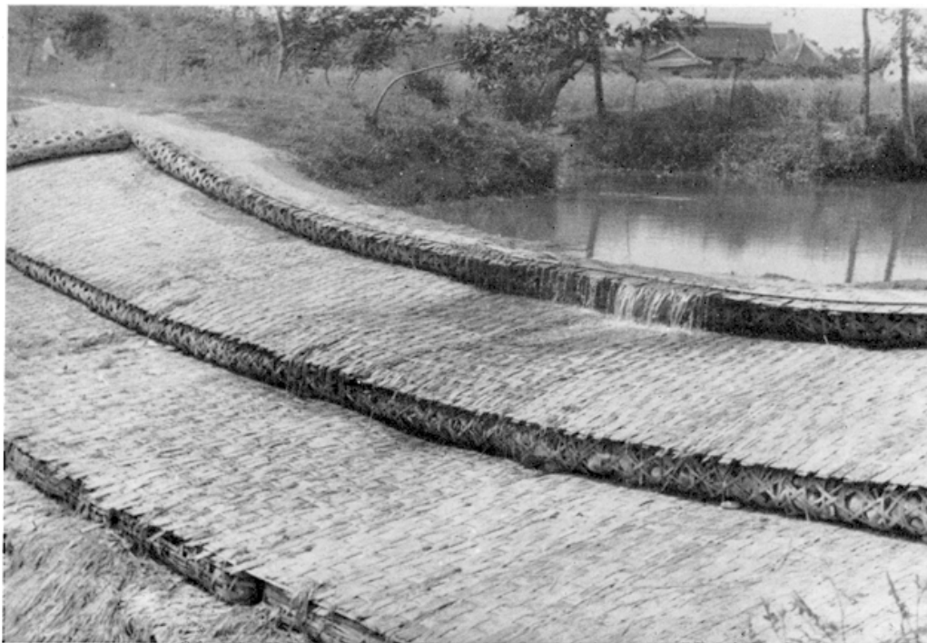
Fig. 913. A weir of gabions near Chhêngtu in Szechuan (orig. photo., 1943). The plaited bamboo cylinders filled with stones can be built into any desired formation; in structures such as this the successive layers are covered with bamboo matting. Cf. pp. 295, 321 ff., 339 ff. and Figs. 895, 914.
