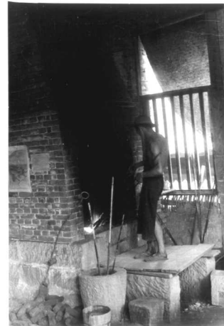
↑ Photograph by Joseph Needham of the operation of a steel-anointing furnace ( mo gang lu 抹鋼爐) at Beibei 北碚 in Chongqing, 1958.
